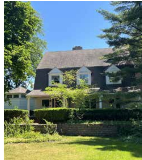
Frank Lloyd Wright's Bagley House
